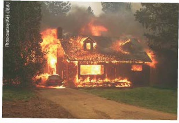
This house was ignited by burning embers landing on vulnerable spots. Notice the adjacent forest is not burning.
