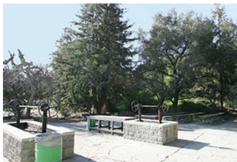
Redwood Glen at Arroyo Verde Park Capacity: 125
