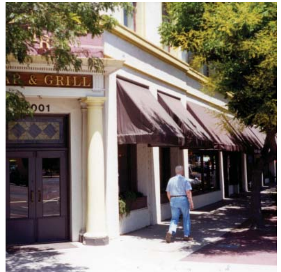
Corner restaurant in Commercial Block building
